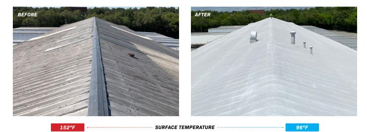
Minimizing the sun's impact on your roof is key to its longevity. The majority of commercial roofing materials are not adequately designed to prevent the flow of heat from constant UV exposure. The Foam-Gard roof restoration system is proven to mitigate the damaging effects of the sun on roof surfaces and effectively reduce interior cooling costs by up to 30%.
