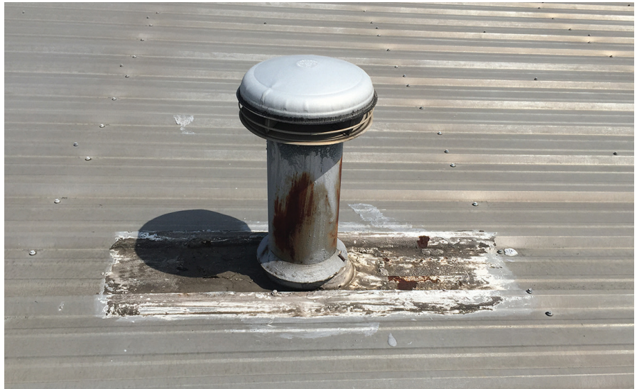
Rusted Penetration
