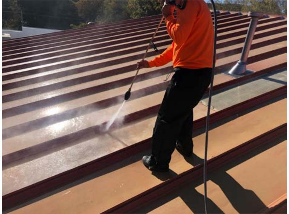
HIGH-TENSILE ACRYLIC 211 APPLIED AS BASE COAT
