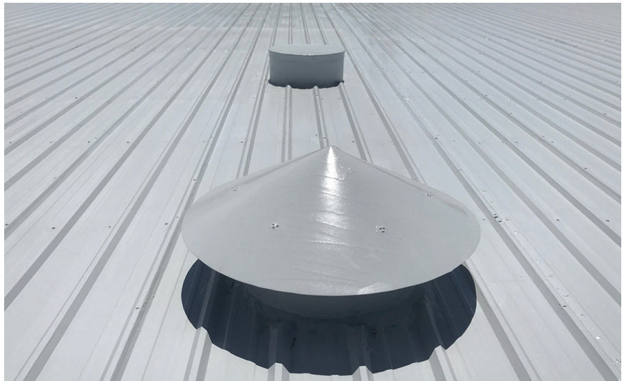
Penetration Detail
